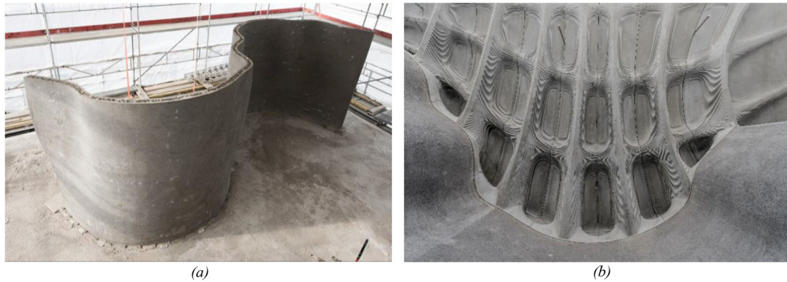
Fig. 26. Mesh Mould wall: (a) after the cover layer was applied (b) after installation of the Smart Slab.
