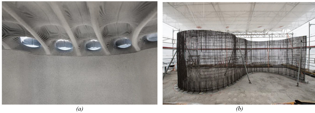
Fig. 22. Structural adaptations: (a) Model close-up of the ribs crossing the wall; (b) final mesh including the additional reinforcement including the compression reinforcement below the crossing points.
