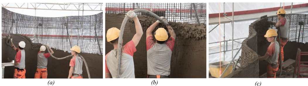
Fig. 23. Filling process: (a) trowelling the freshly filled mesh; (b) close-up of the filling process showing the un-trowelled concrete; (c) filling the upper region of the mesh.
