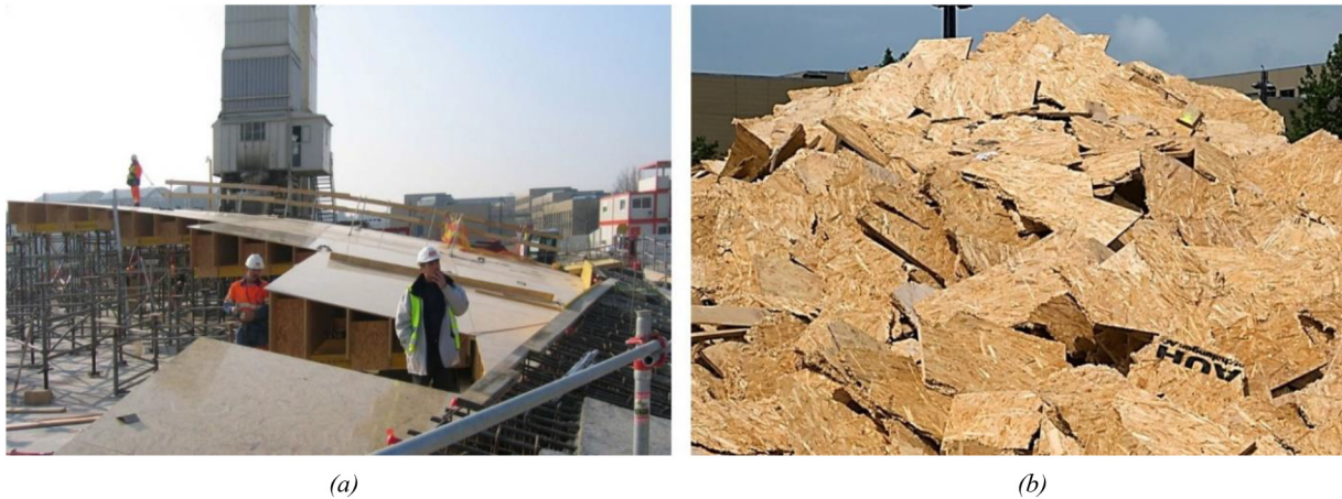
Fig. 2. EPFL Rolex Learning Center construction process: (a) installation of the unique formwork tables; (b) construction waste after stripping the formwork.
